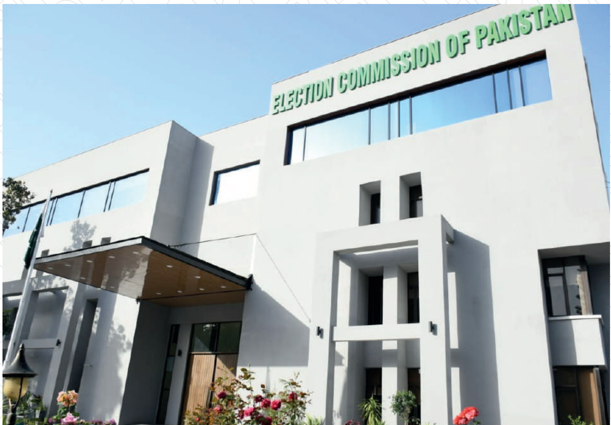
Uplifting of Front Facade of ECP building at Islamabad Secretariat
